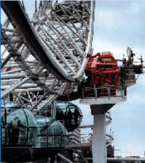
Rexroth played a major role in equipping the "London Eye" built for the millennium celebrations. It supplied the drive, the electronic controls and the anchoring and stabilizing system.
