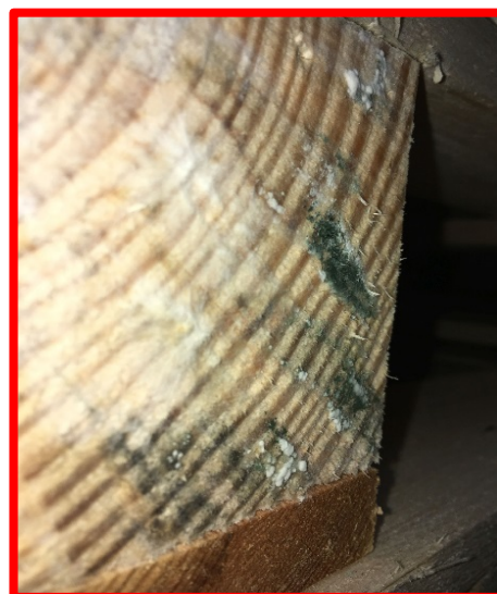
Figure 20: not ok, mould, sponge, dry rot
