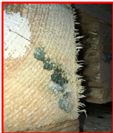
Figure 15: not ok, mould, sponge, dry rot
